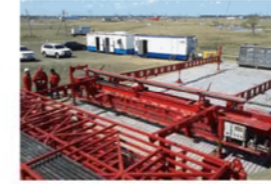
Onsite application of hydraulic pipe box (Pipe in)
