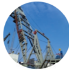
8000m Swing-up drilling rig
