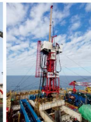
SDYJ225 on offshore platform
