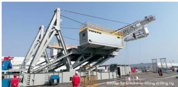
8000m Synchronous-lifting drilling rig
